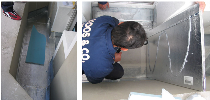
▲ Building renovation in Vienna: Glue on the VIP
