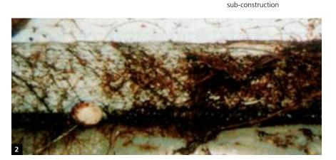
Mechanical stresses on the waterproofing caused by the pavement and the traffic load
