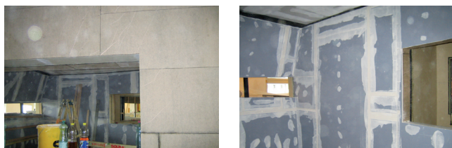
Construction of a broadcasting studio with Idikell® heavy foils
